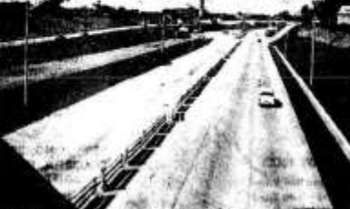
Interchange at Evans and Northwest Expressway. On modern concrete highways like these, speed can stay low. Add the 50 year life engineers can design into concrete and figure some real big savings!
