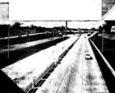
Interchange at Evans and Northwest Expressway. On modern concrete highways like these, speed limits stay low. Add the 50 year life engineers can design into concrete and figure some real big savings!
